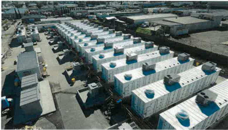
Figure 4: Example of a Lithium-Ion BESS installation
